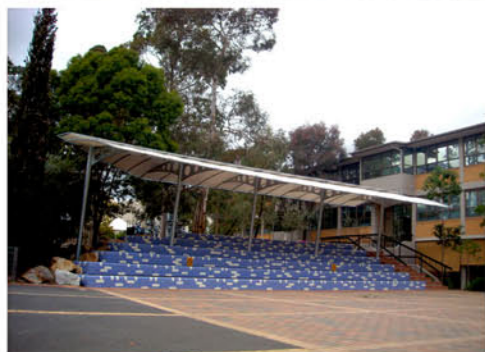
Extensive Landscape Works 1996-2010 Primary Library School Piazza
