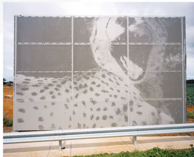
Punched metal freeway signage screens
