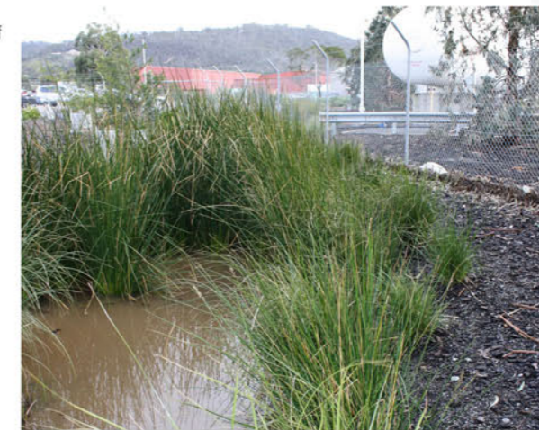
Storm water catchment and filtration swale
