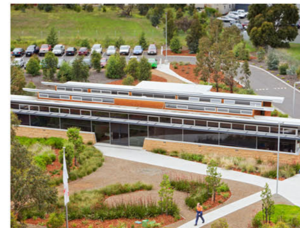
Administration Office Landscape courtyard
