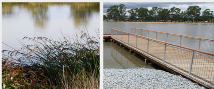
Victoria Park Lake redevelopment, Shepparton
